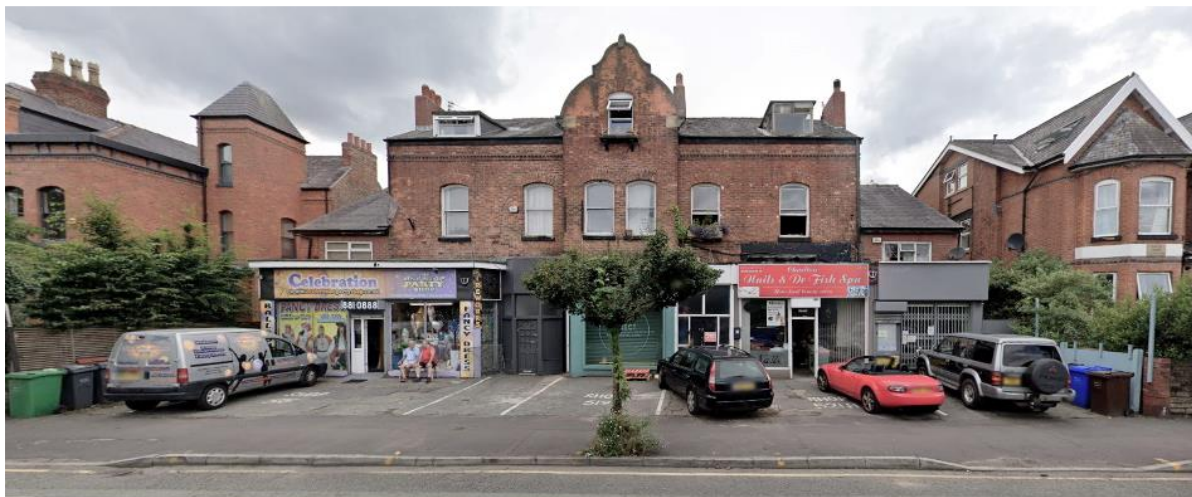
Front elevation from Barlow Moor Road
